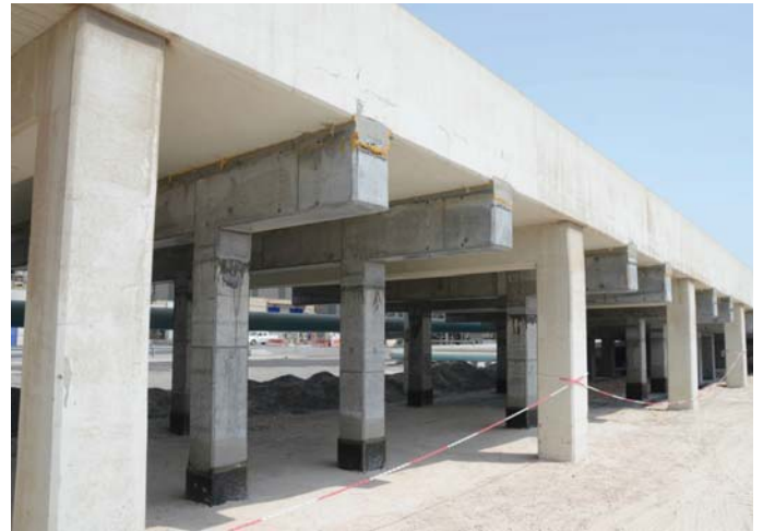
Strengthened ramp supports in grey concrete
